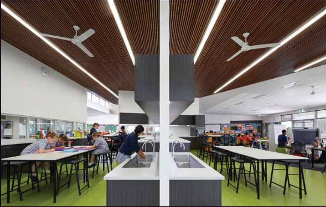
surface mounted continuous linear LED strip lighting in aluminum channels flat and bright for 4m high ceiling
