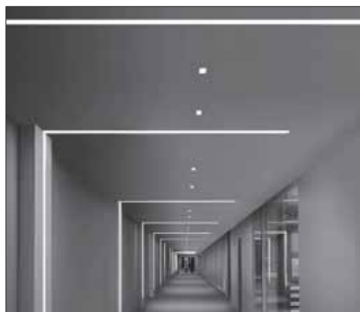
recessed continuous LED lighting mounted into walls and ceiling decorative and functional
