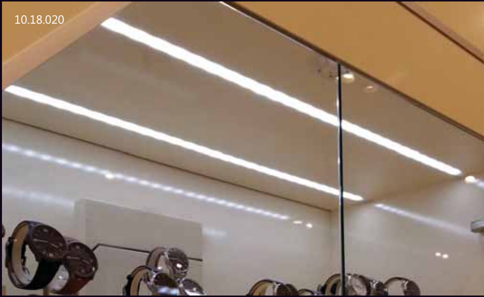
recessed linear LED lights for under-shelf lighting flat and slim
